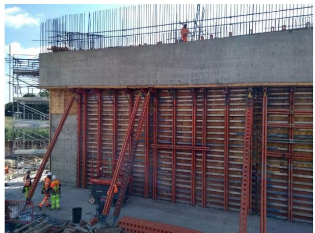
The Central Pier of the Bridge is the last part of this phase of the works before the main bridge columns are constructed. The steel structure of the bridge columns have been formed off line and are being moved into place.
